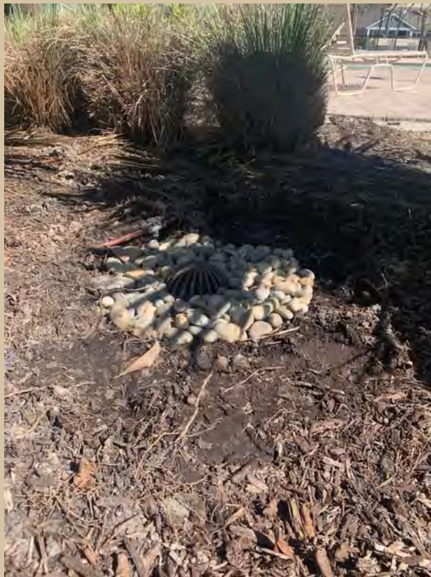
ROCKS INSTALLED TO PROTECT DRAINAGE
